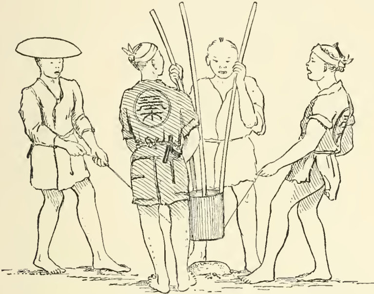
FIG. 5. — POUNDING DOWN FOUNDATION STONES.
